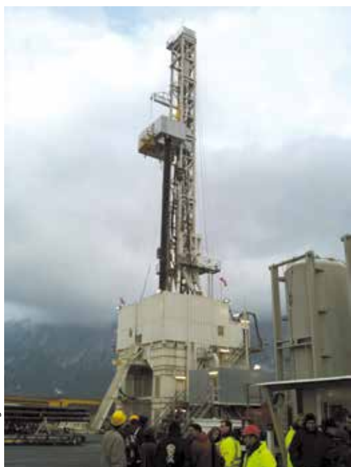
Figure 4 Tour de forage Noville 2010.
